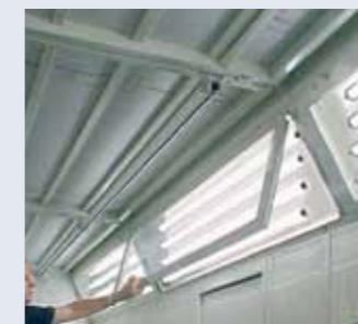
Hinged light fixtures for ease of cleaning and maintenance.
